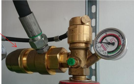
The pressure controller allows for a reduction of the overpressure peak during the discharge.
